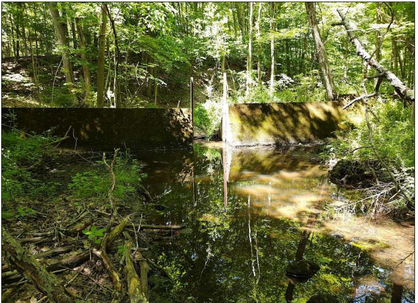
Figure 41. Looking north at the water gap showing center sections of the dam and the vertical steel posts that were once part of a sluice gate.
