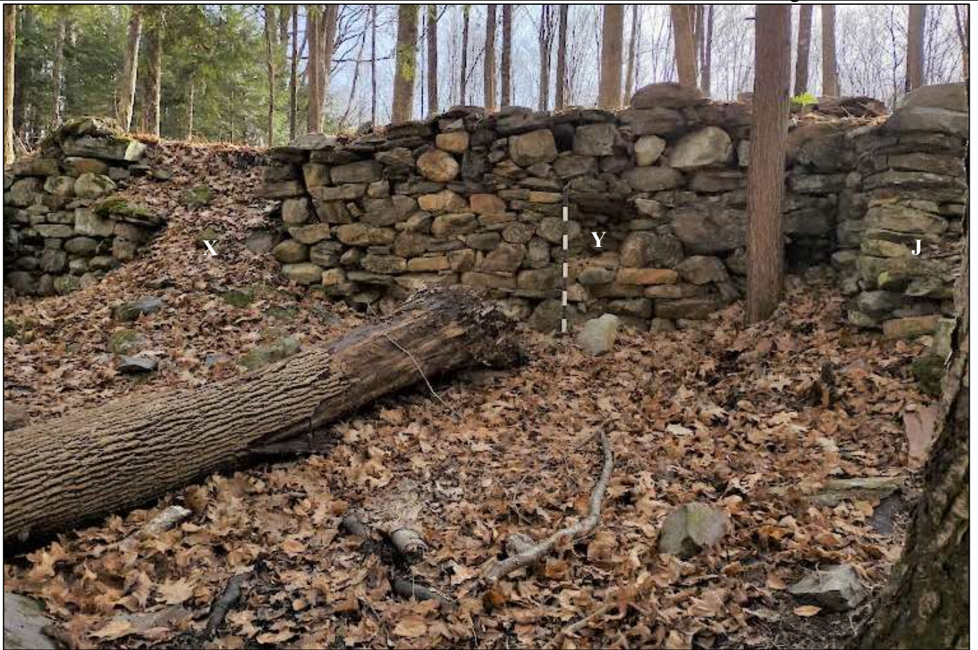
Figure 65. Looking southeast at Wall E. At the left edge of the photo is the junction of Wall E and Wall D. At the right edge of the photo is the junction of Wall E and Wall J. A large disturbed area is marked with an X. A smaller area where stones have fallen out or were deliberately made into a niche (labeled Y) is visible to the right of the 1-meter stadia rod.
