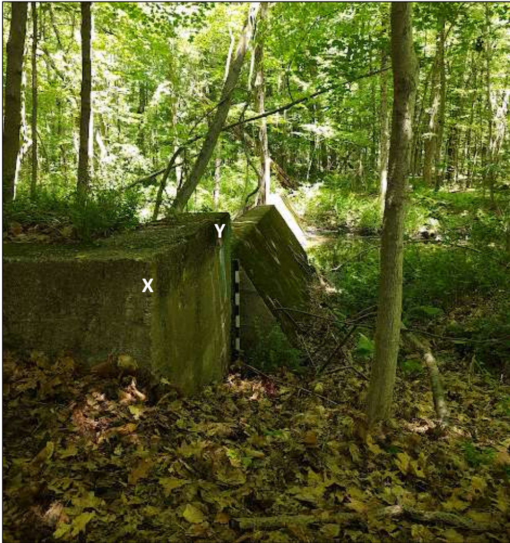
Figure 38. Looking east-northeast at the outside of the southwest corner of the dam (marked with X). The photo shows that the outside of the corner is well above ground level (28 inches), while the inside is at ground level. At point Y, the wall is four feet 8 inches high.
