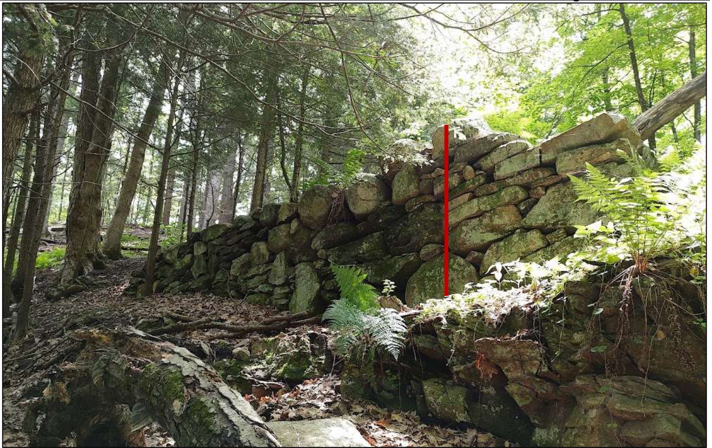
Figure 71. Looking south-southeast at the north side of Wall K. The complete 28-foot length of the wall is visible. The vertical red line is 75 inches, the maximum height of the wall.
