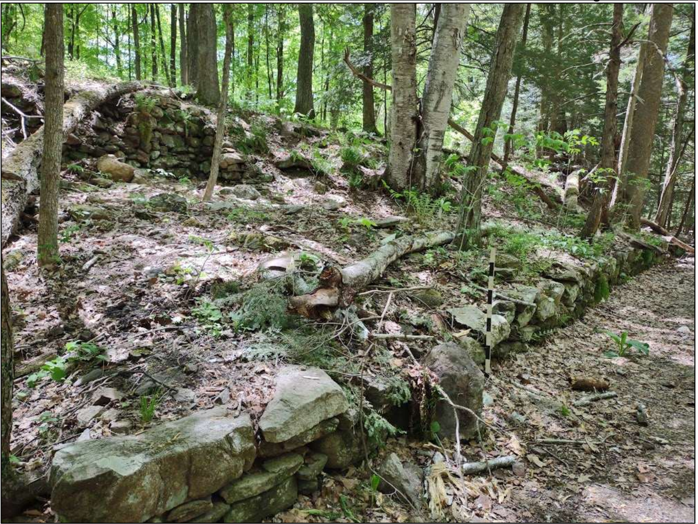
Figure 75. Looking southwest at a piece of Wall A that was recently damaged when a large branch from the birch tree in the background fell on it.
