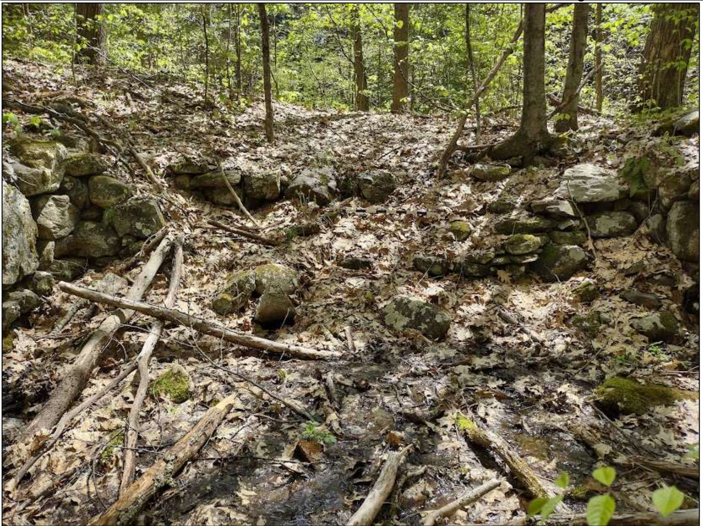
Figure 99. Looking south at the south wall of the East Section. The middle is deteriorated while the east and west ends retain more integrity. A lower wall appears to be backed by a higher wall.
