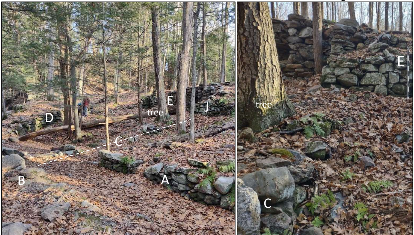
Figure 60. Walls C and J are indicated to illustrate the difference in height, integrity, and solidity. The dashed line in the left photo follows the line of Wall C and shows that much of the wall has very little integrity or visibility. In the left photo, the less substantial quality of Wall C compared to Walls B, D, E, G, and J is illustrated. In the right photo, a relatively intact portion of Wall C is in the lower left corner under a tree that is labeled in both photos.
