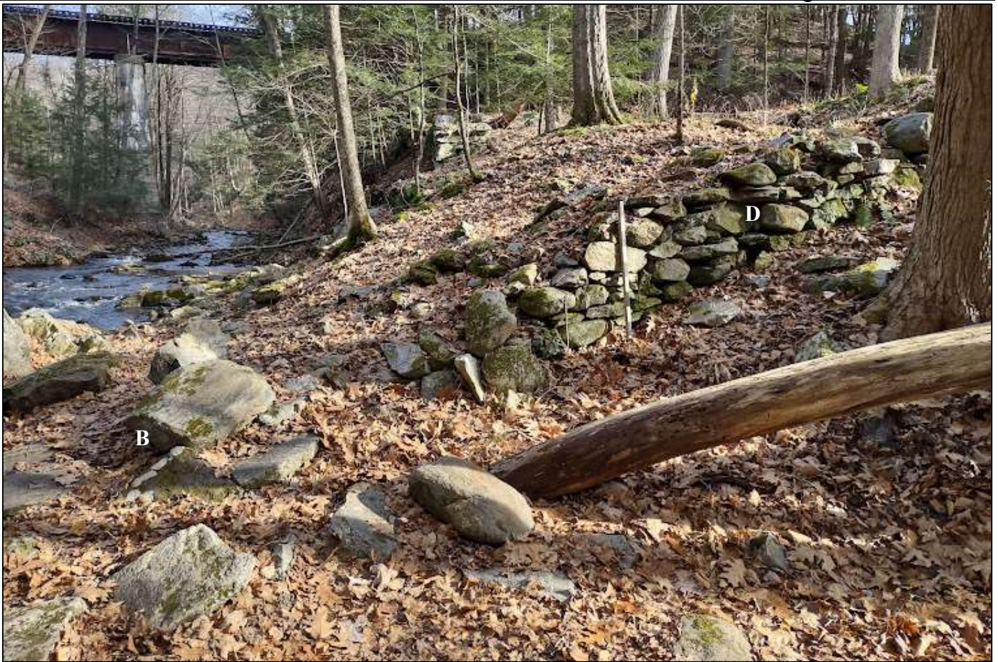
Figure 64. Looking east at the northern end of Wall D and the eastern end of Wall B. Both walls are badly deteriorated here, probably as a result of river action, although it is possible that upheaval of trees along the riverbank may have been responsible.
