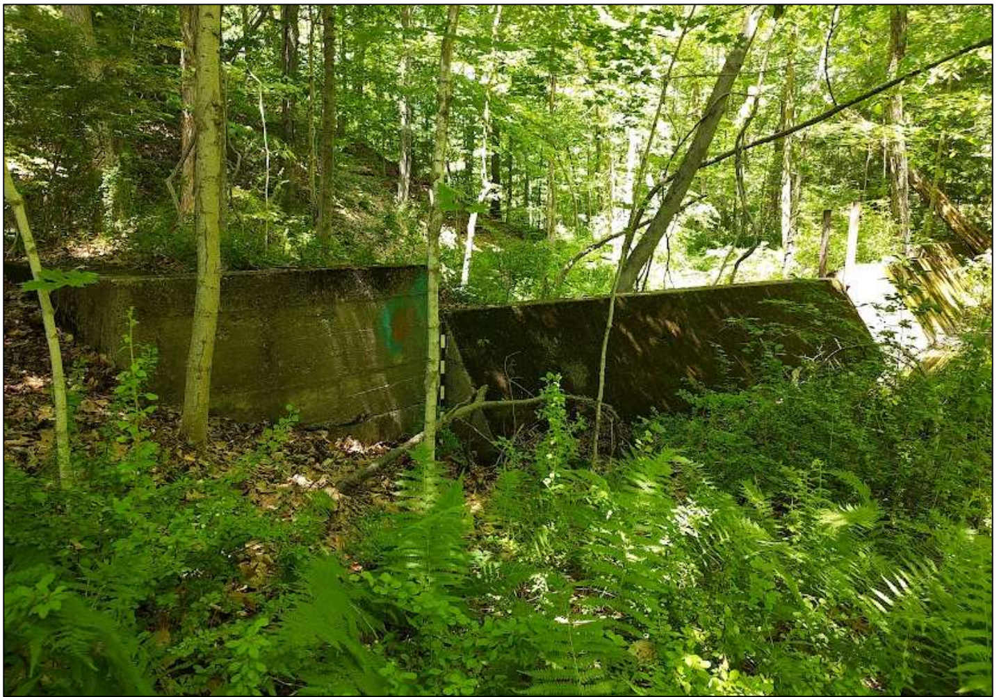
Figure 39. Looking northeast at the west and west-central sections of the dam illustrating the 14-inch change in wall height (obscured by the tree just left of the measuring stick). There is also an example of graffiti to the left of the tree.
