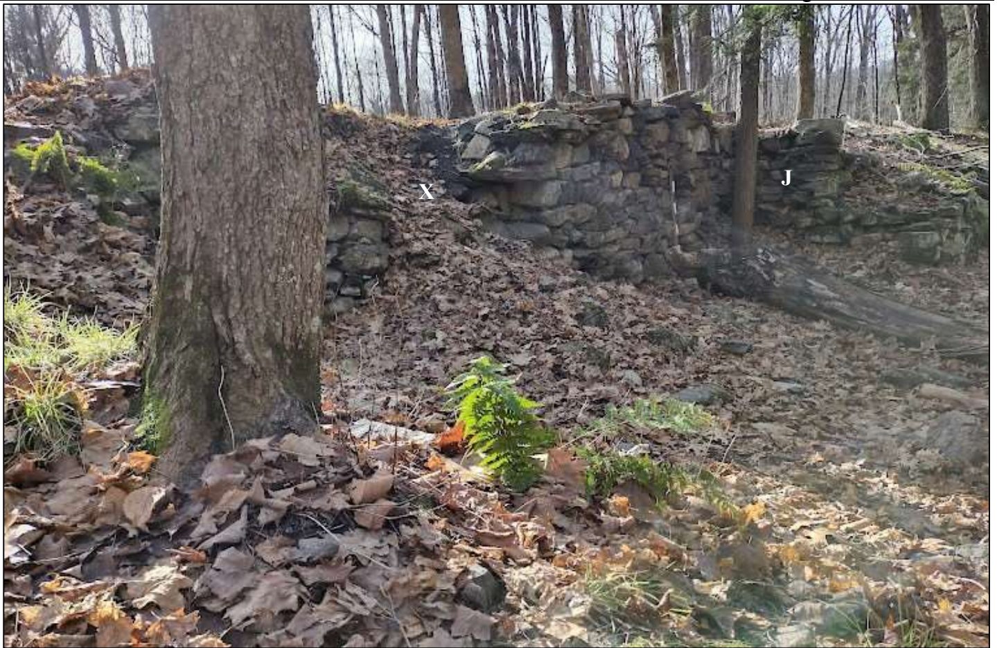
Figure 66. Looking southwest at Wall E and the junction of Wall E and Wall J (Wall J is, appropriately, labeled with a J). The large disturbed section shown in Figure 20 is again marked with an X. The 1-meter stadia rod is in the same position as in Figure 20.
